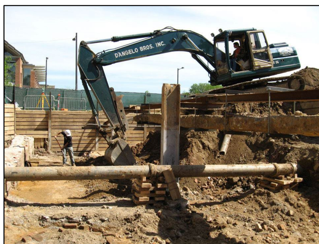
Construction equipment bulk excavating fill from within the excavation area.
