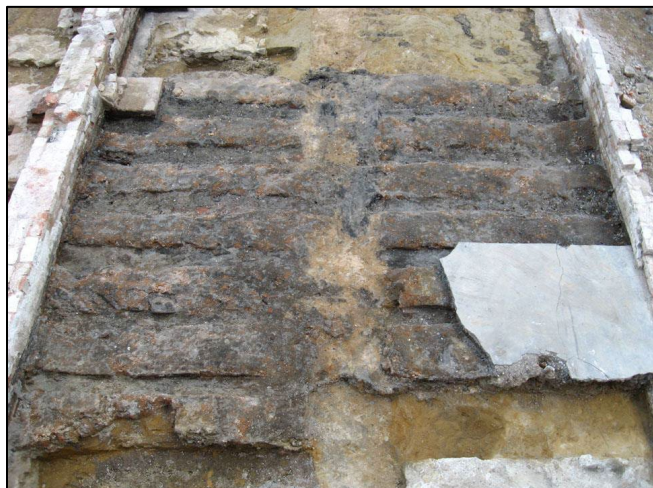
An overview of the nineteenth-century basement floor level (Lot 528). The parallel depressions in the floor are from the floor joists, now decayed. The small flat gray section to the right is a remnant of the overlying twentieth-century cement floor.
