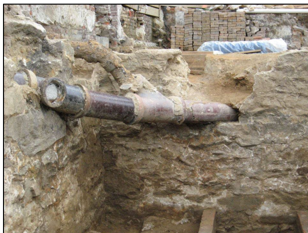
The construction of this terra-cotta drainpipe required upper portions of the root cellar walls to be removed.
