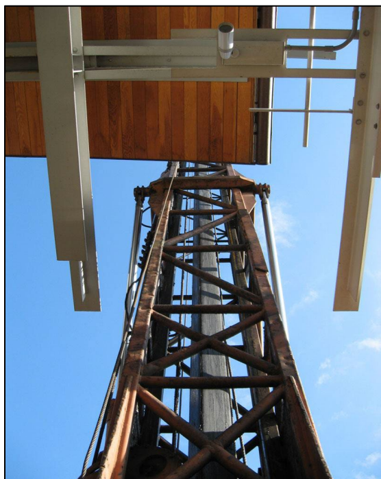
Drilling for soldier piles in front of the Liberty Bell Center.
