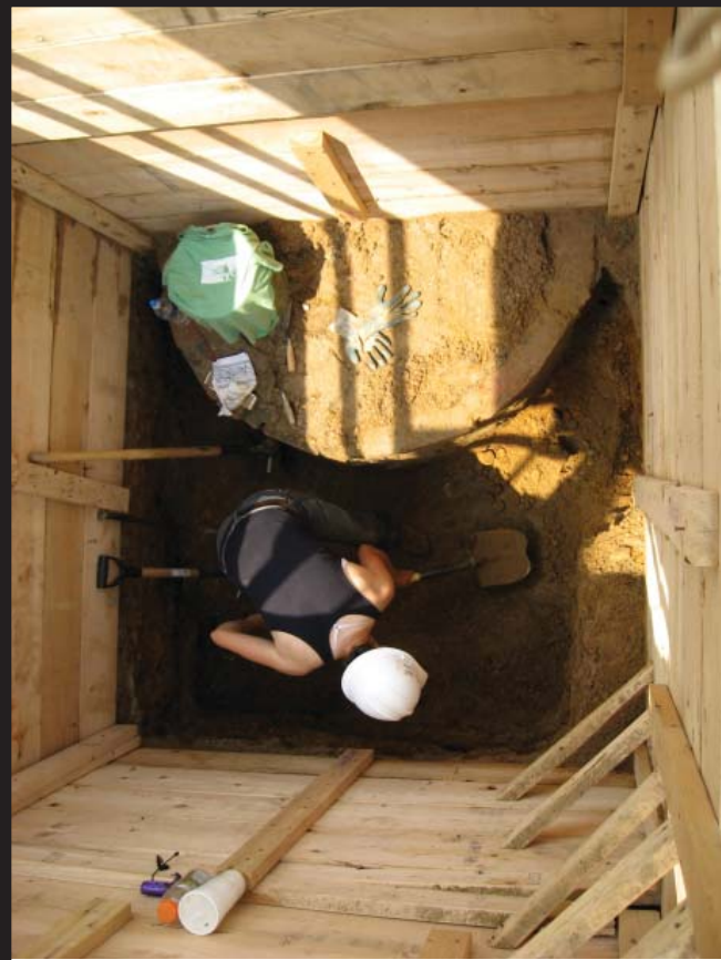
Bisecting the shaft within the shoring box
