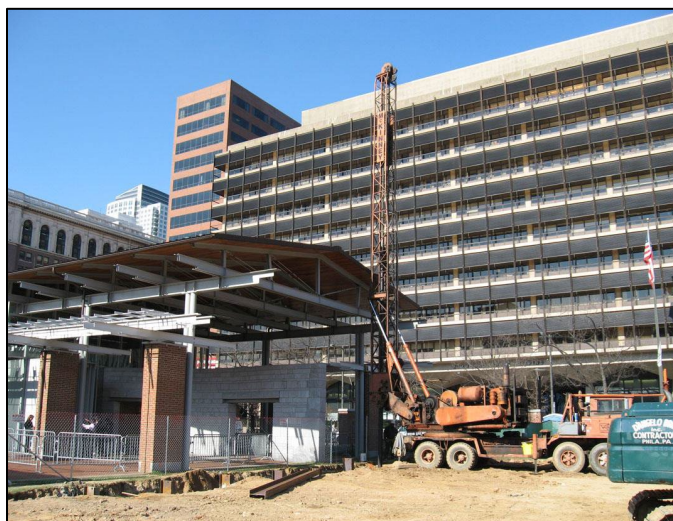
Drilling for soldier piles in front of the Liberty Bell Center.
