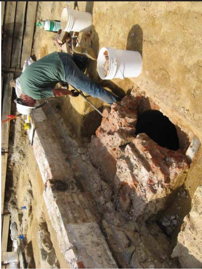
Dismantling the brick cap and the empty upper part of the shaft below
