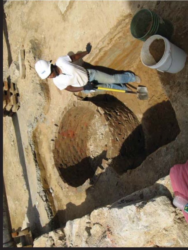
Exposing the shaft and getting ready to install the shoring box
