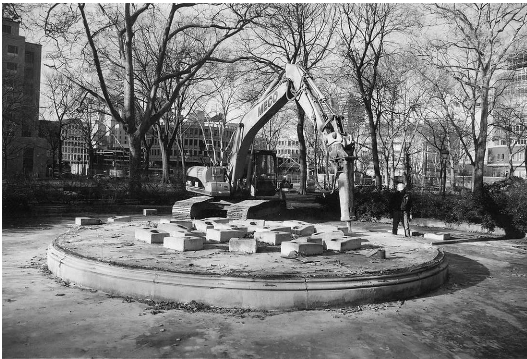
Plate 2. Demolition of fountain interior, view southwest.
