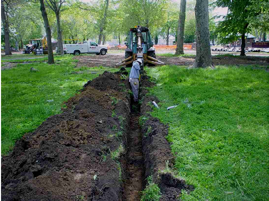
Plate 11. Excavation of Trench 10 in progress, note clean subsoil fill, view southeast.
