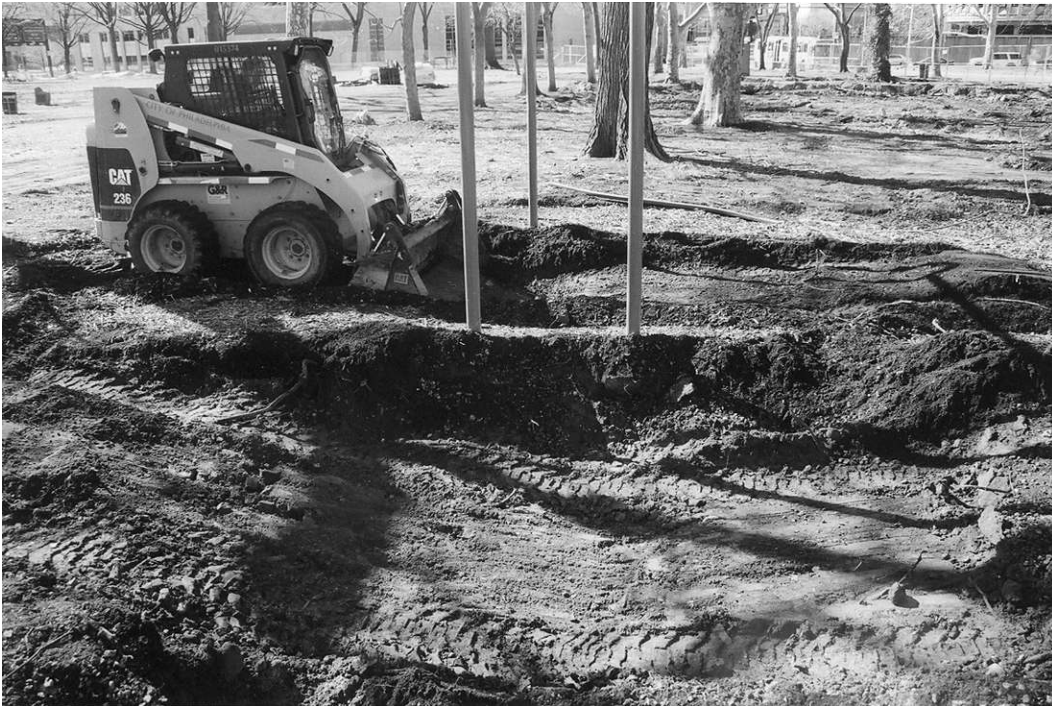
Plate 8. Demolition of swings with clamshell bucket, view south-southeast.
