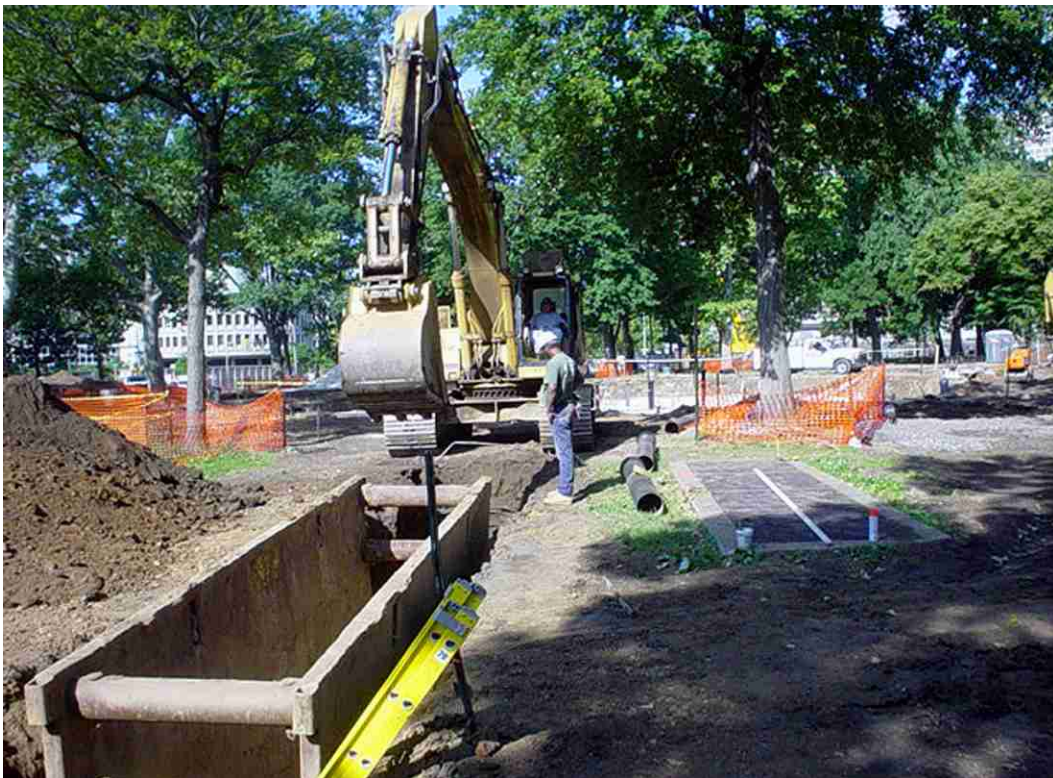
Plate 17. Trench 19A general view, note PATCO vent to right, view west-southwest.
