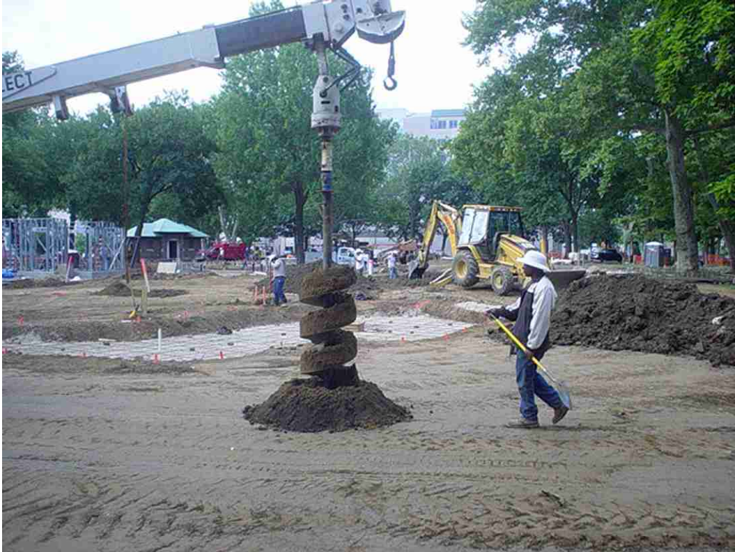
Plate 43. Excavation of AT 19, view south.
