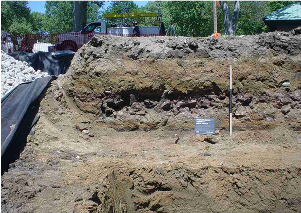
Plate 14. MH 1 at west end of Trench 13, north profile, view north, note seepage bed at left.
