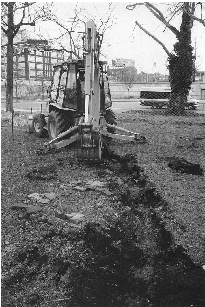
Plate 5. Demolition of serpentine brick coping, view northeast.
