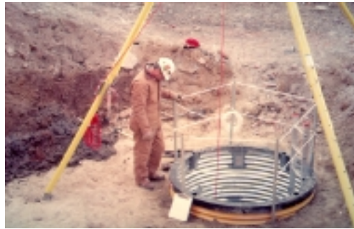
Beginning Excavation of a Deep Well.
