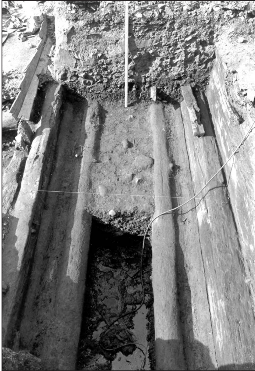
Figure 43. The initial discovery of the slipway.
