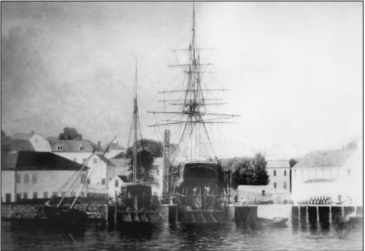
Figure 84. Three masted on the Gloucester Railway. Lane, 1857.
