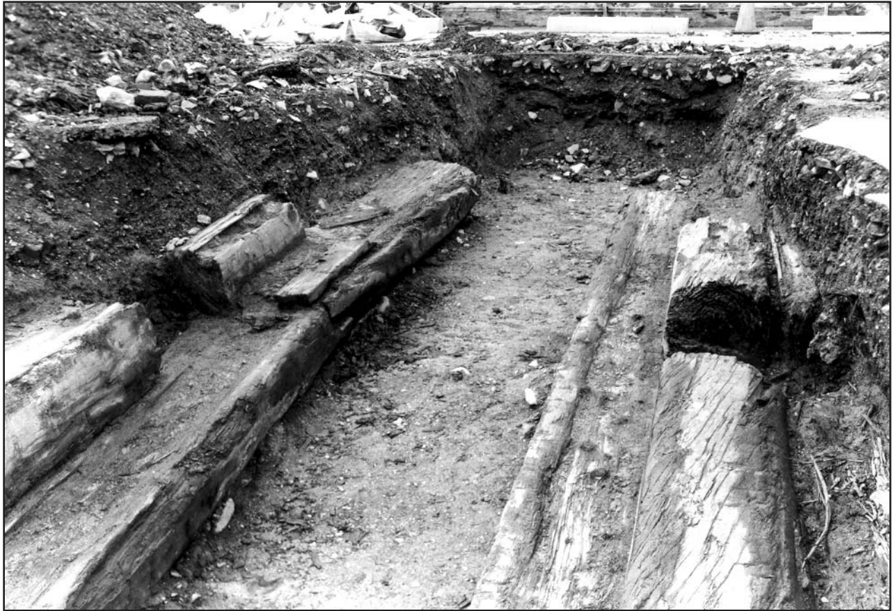
Figure 49. HAER photograph of the shore end of the slipway. View west.
