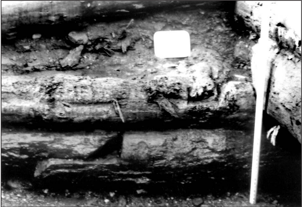
Figure 34. Circa 1760s wharf, Test Trench #1, west wall.
