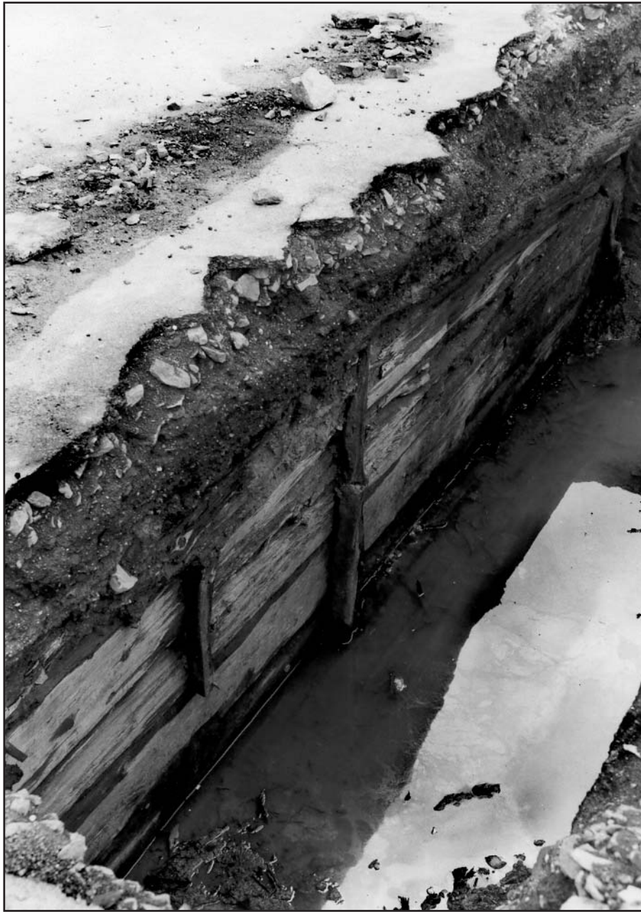
Figure 66. Nineteenth-century wharf bulkhead, Test Trench #7. View northeast.
