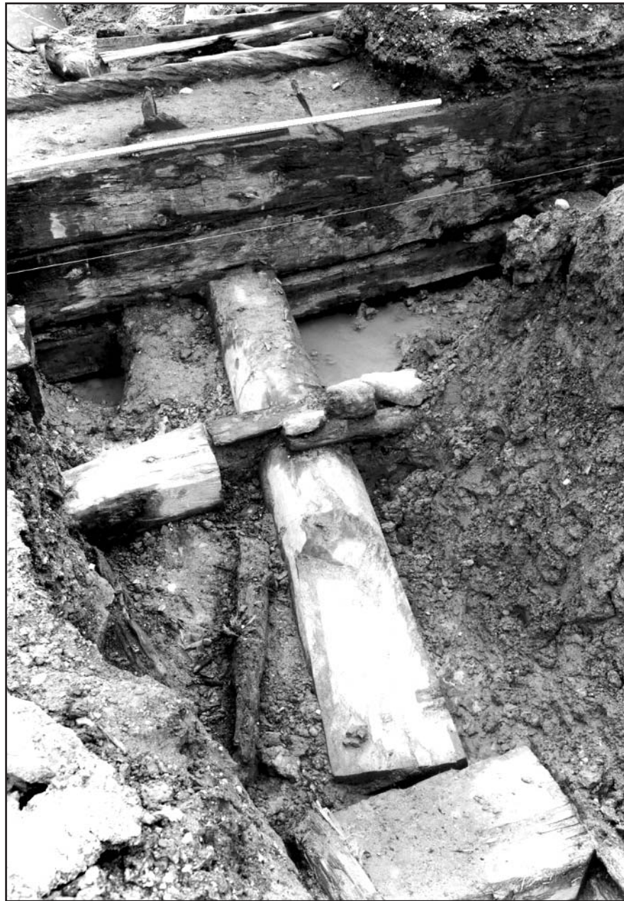
Figure 74. HAER photograph of Test Trench #6. View south.
