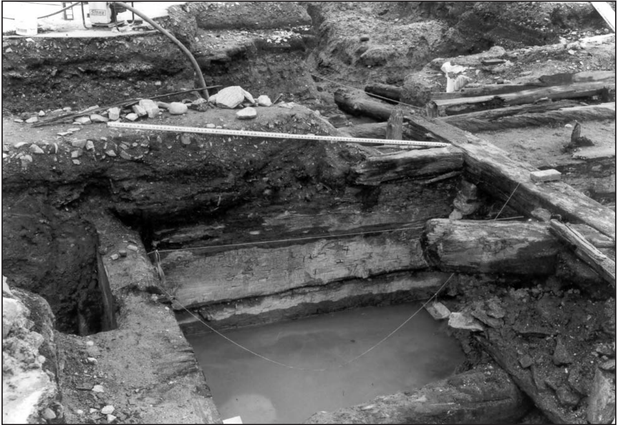
Figure 64. HAER photograph of Test Trench #11 and ER #33.
