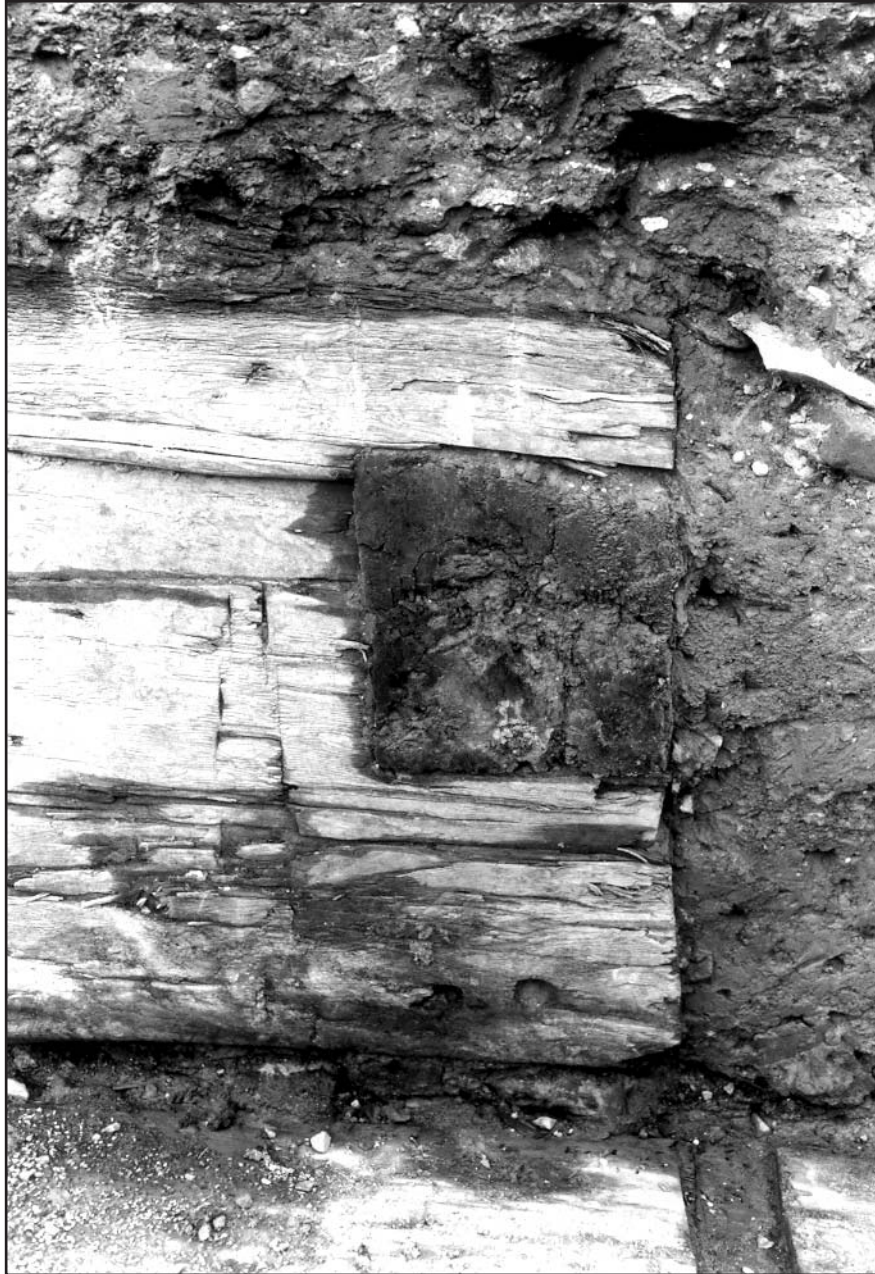
Figure 48. Photograph of the river end of Feature #14. View north.
