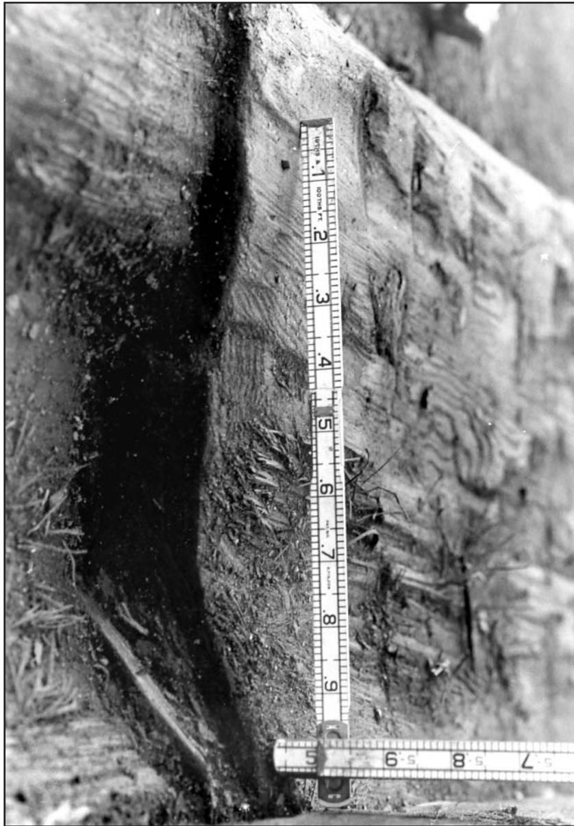
Figure 52. Close-up photograph of the slipway track.
