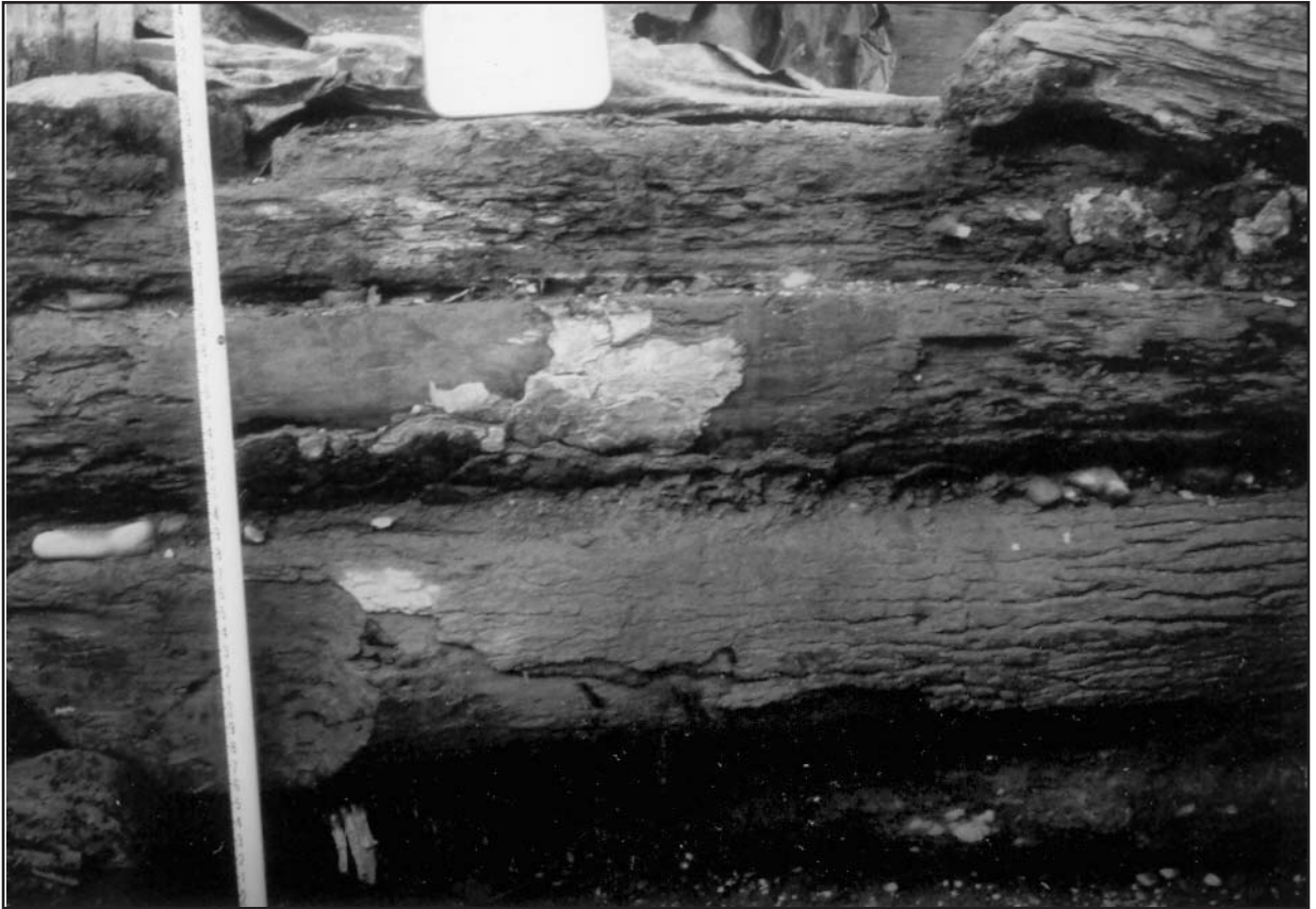
Figure 37. Photograph of the interior of the late eighteenth-century wharf bulkhead. View north.
