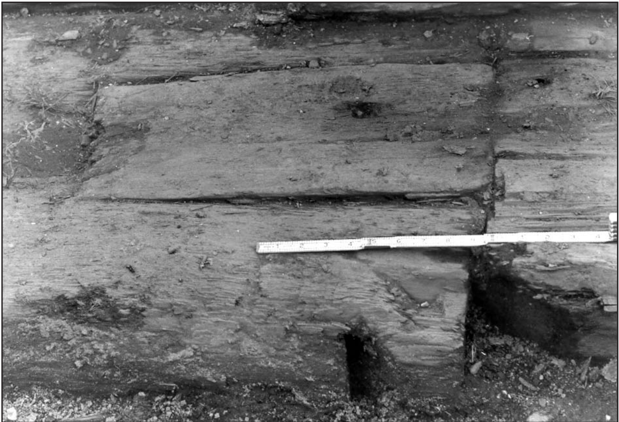
Figure 55. Repair of the slipway track, southern running way.
