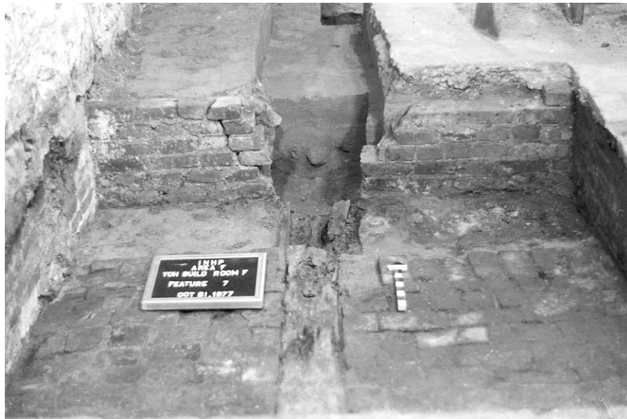
Plate 28. Area F, Yoh Building, Room F, showing the wooden beam of Feature 7 anchored in the center of the feature.
