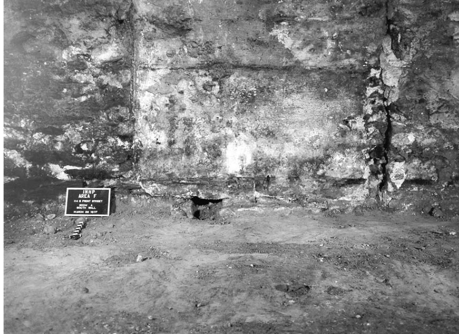
Plate 31. Area F, 114 S. Front Street, Room A; arrow points to vertical joint in south wall. Note void of former floor joist in south wall.
