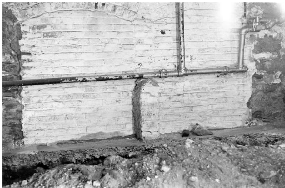
Plate 6. Area F, Yoh Building, Room B; west wall. Note closure of arched openings to Second Street; view west.
