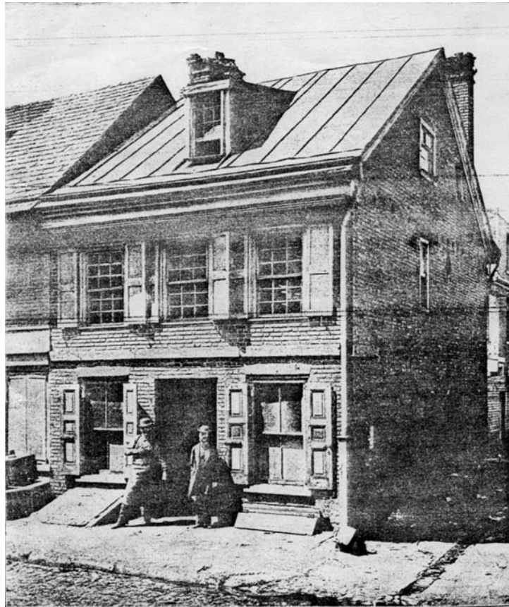
Figure 33. The Letitia Penn house built on Letitia Court c.1713, a short distance from Morris Alley, that fits the description of the house built by Anthony Morris c.1688 on Front Street. The top view is a drawing of the house from Watson 1870 and the lower view is a nineteenth-century photograph of the house.
