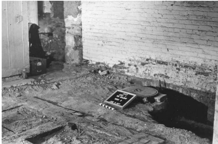
Plate 7. Area F, Yoh Building, Room B; east wall. Note brick arch opening into Room C, manhole cover of Feature 1 right center, and brick foundations for a furnace/boiler (Feature 2) in the foreground; view northeast.
