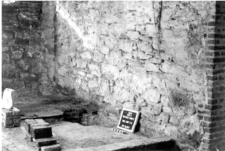
Plate 21. Area F, Yoh Building, Room F, wall unit P-Q, view southwest. This stone wall may be the west wall of 1-3 Gray's Alley. The brick facing at the right was added when the wall was broken through to create a door opening in the later warehouse.
