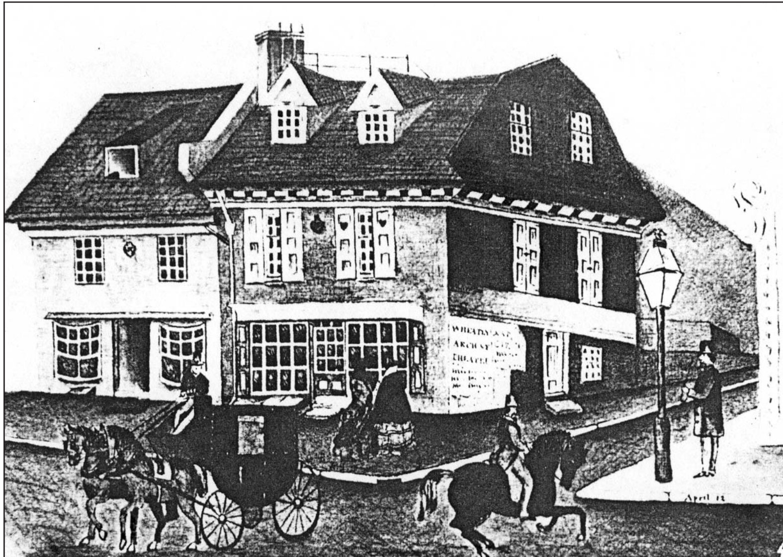
Figure 8. Undated watercolor of 77 and 79 South Second Street (Green :112). The corner house (79 later 123) with the gambrel roof, occupied by sea captain Stephen Anthony, was the third to be built (c.1692) on the Area F site. The house next door (77 later 121) was built next c.1697.
