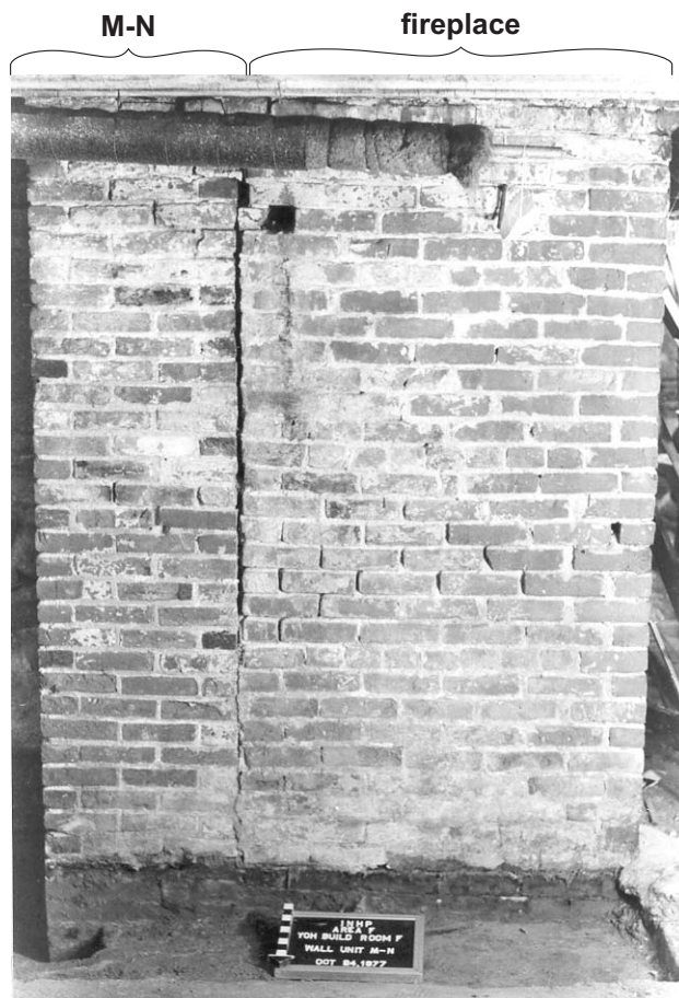
Plate 18. Area F, Yoh Building, Room F, wall unit M-N; view south. The seam shows the finished brick end of wall L-M and added brick chimney at right.
