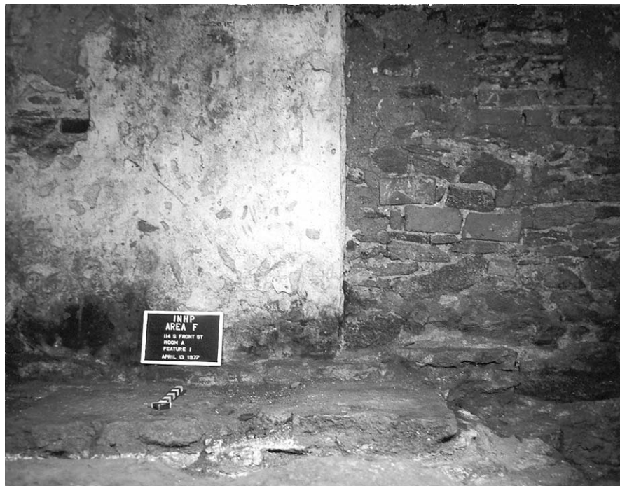
Plate 34. Area F. 114 S. Front Street, Room A, Feature 1, c.1856 floor remnant in southeast corner of room; view south.
