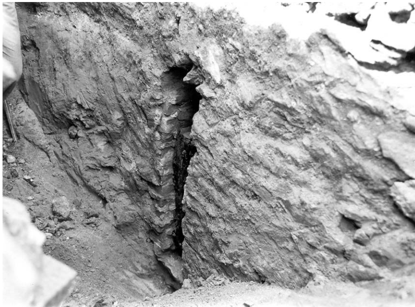
Plate 44. 116 S. Front Street, vertical pocket in foundation wall after removal of wood; view north.
