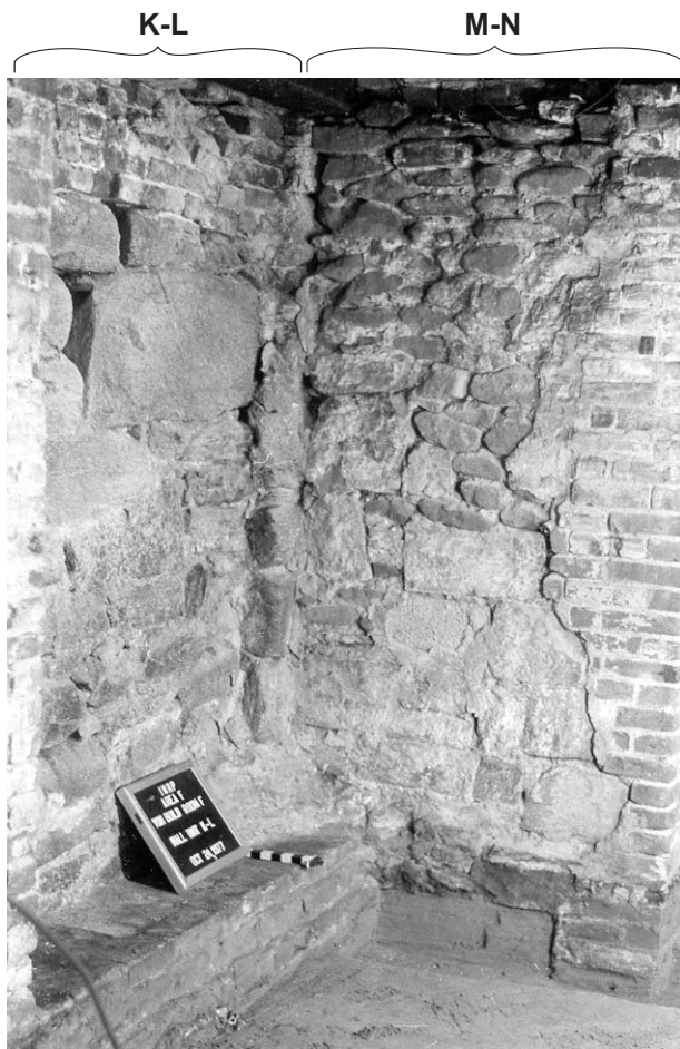
Plate 17. Area F, Yoh Building, Room F, southwest corner, wall units K-L and L-M; view southwest. Note filled in doorway at left and brick facing, right, added to finish edge of truncated wall L-M.
