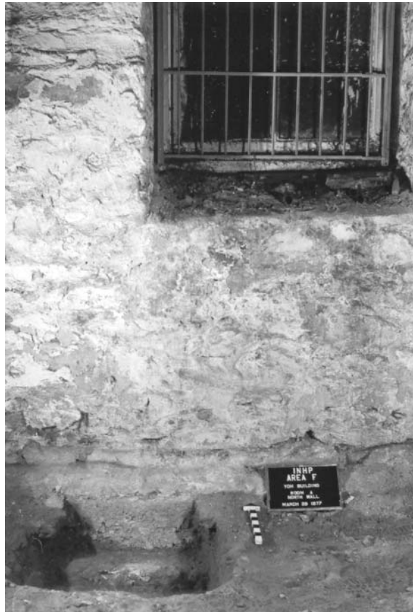
Plate 1. Area F, Yoh Building, Room A; north cellar wall showing one of the three windows along this wall.
