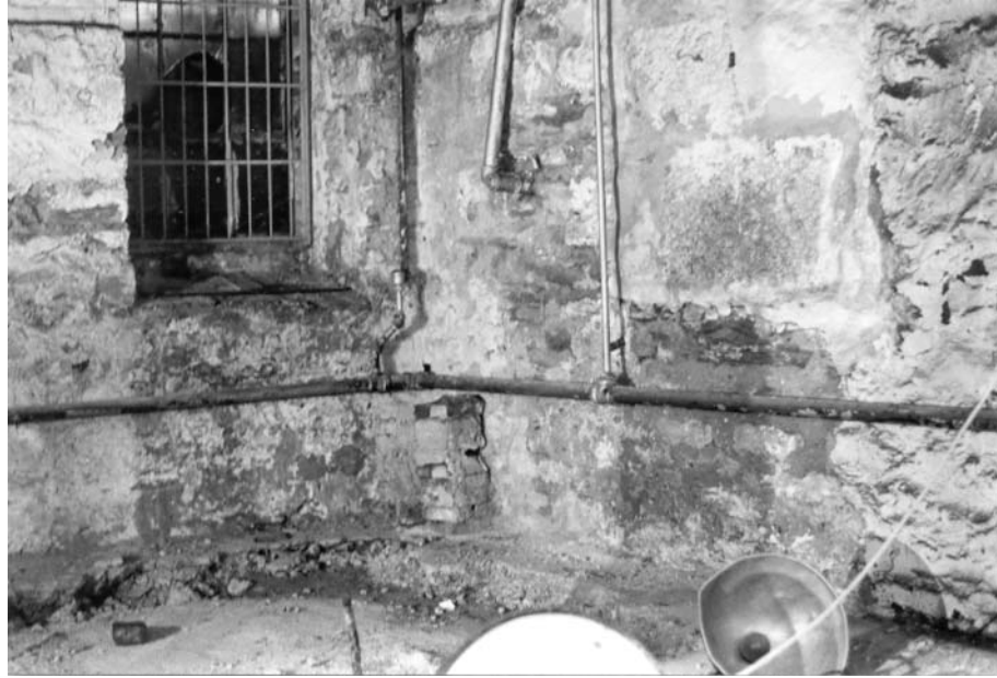
Plate 5. Area F, Yoh Building, Room B; southwest corner. Note closure of opening in west wall; view southwest.
