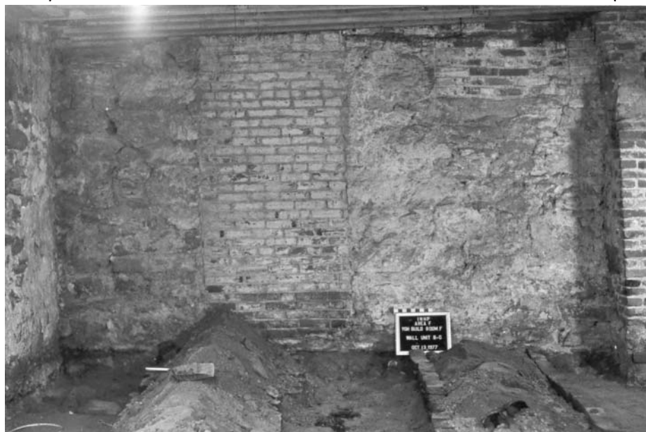
Plate 14. Area F, Yoh Building, Room F, wall unit B-C, shared west wall of Room C, 114 S. Front Street. Note brick sealing former door connecting brick store with rear warehouse c.1847.
