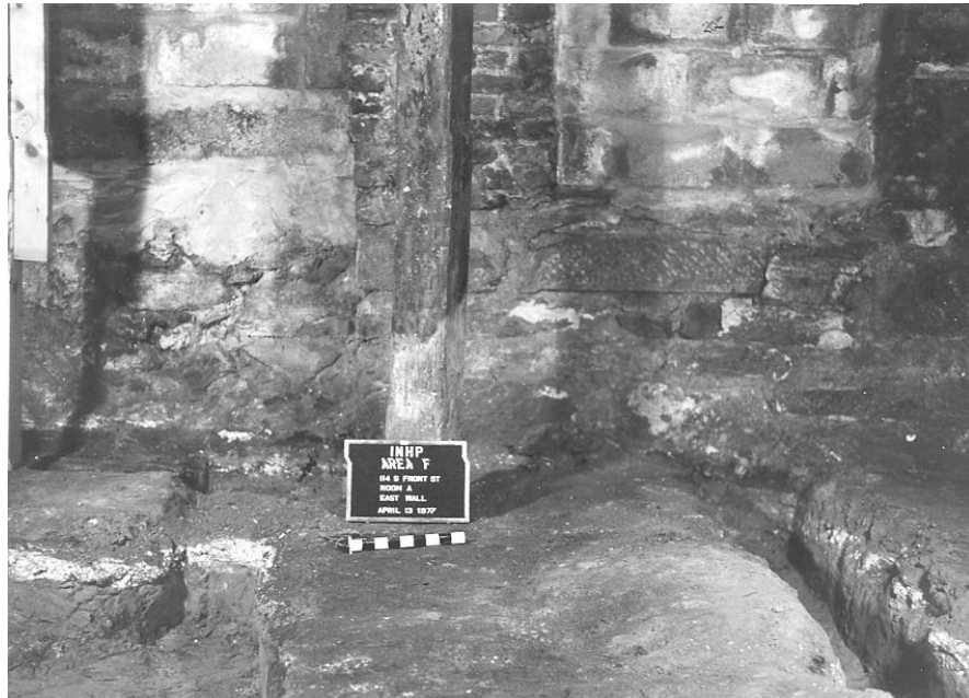
Plate 33. Area F, 114 S. Front Street, Room A, east wall. Note structural changes in east wall and lime mortar in basement floor.
