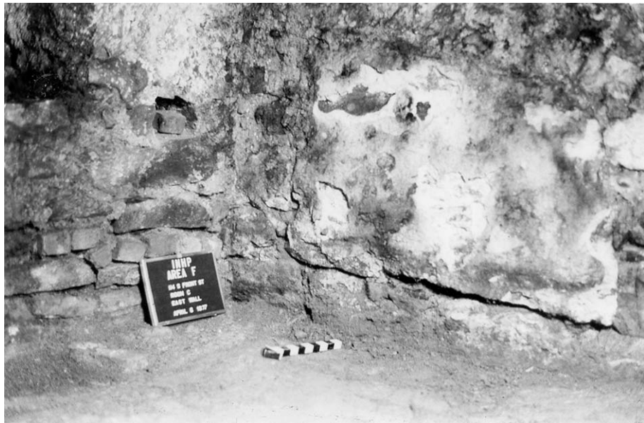
Plate 41. Area F, 114 S. Front Street, east wall. Note brick patch in wall.
